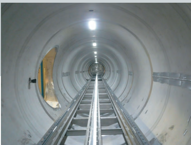
Inside view of the 34 m detector tube at ID02. The detector wagon at the far end travels along the rails.
